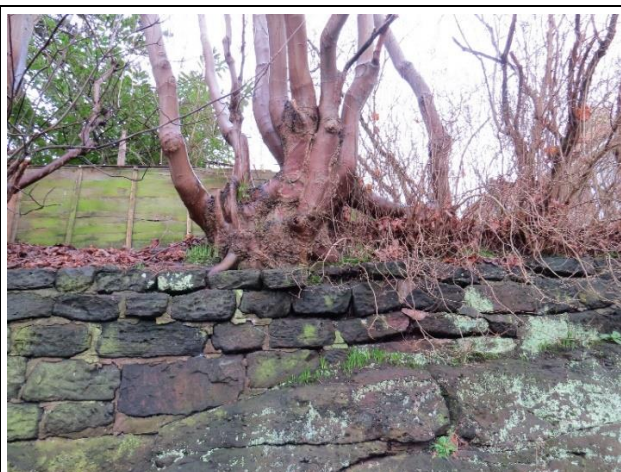
Stone Wall Incorporating Bedrock
