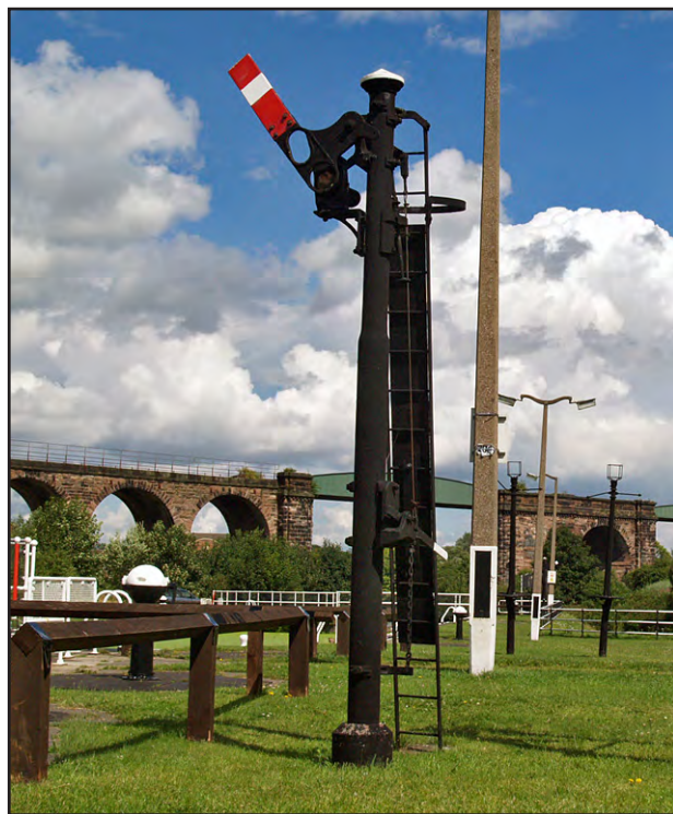
Fig 88: Former railway signals protecting the locks at Hunts Lock on the River Weaver Navigation © David Ingham 2008. Used under the Creative Commons Attribution-Share Alike 2.0 Generic licence.
