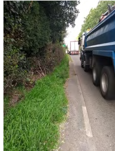
FIGURE 7: HGVs ON THE A51 THROUGH CLOTTON. PAVEMENT SEVERELY OVERGROWN
