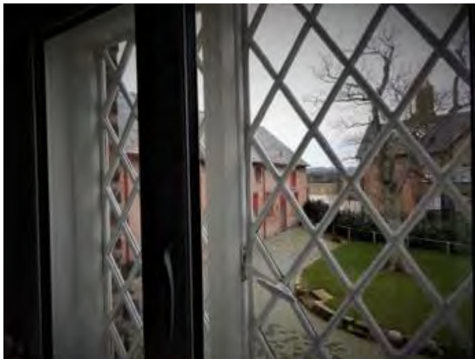
FIGURE 12: ORIGINAL HERITAGE WINDOWS RESTORED
