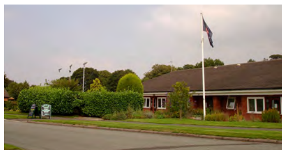
Delamere Park Clubhouse
